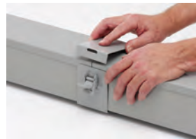
Install outside connector around wireway splice location
