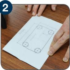
Once measured, place the installation template on the floor and cut a hole accordingly. A small drill, jigsaw, or hole saw can be used to precisely cut the hole required.
