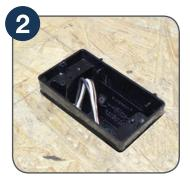
Move floor box in highest position by loosening slider plate screws, install sub floor around raised box
