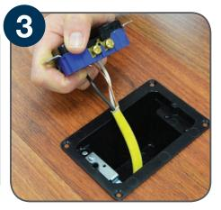
Bring the electrical cable through the preferred box clamp, and place the box down in the hole and secure it with the preferred mounting method. Wire the device according to local electrical code.
