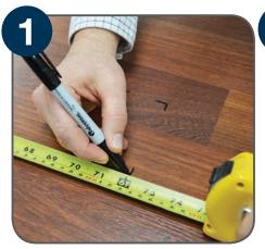
Find a location in between floor joists and measure the box dimensions according to the template supplied in the installation instruction sheet.
