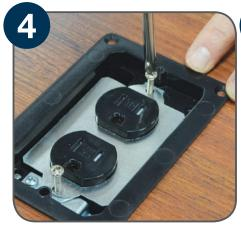
Once the device has been wired, secure the device and dust plate down into the box using the screws supplied in the packaging.
