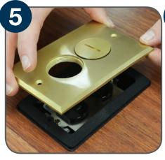
Place the cover gasket on the box flange and position the cover assembly over the gasket to ensure an adequate seal between box and lid is met.
