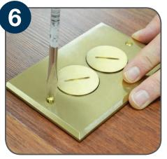
Secure the cover to the box with the screws supplied in the packaging. Attach all screw plugs and keystone plugs as required.
