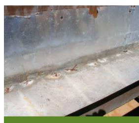
Pressure treated wood will corrode aluminum and galvanized flashings
