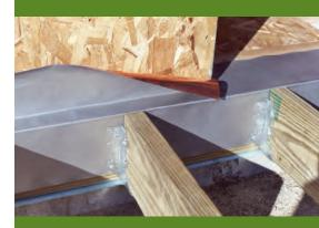
YorkShield 106 PT copper flashing will not corrode when in contact with woods designed for ground contact treatments provided a lifetime flashing solution.
