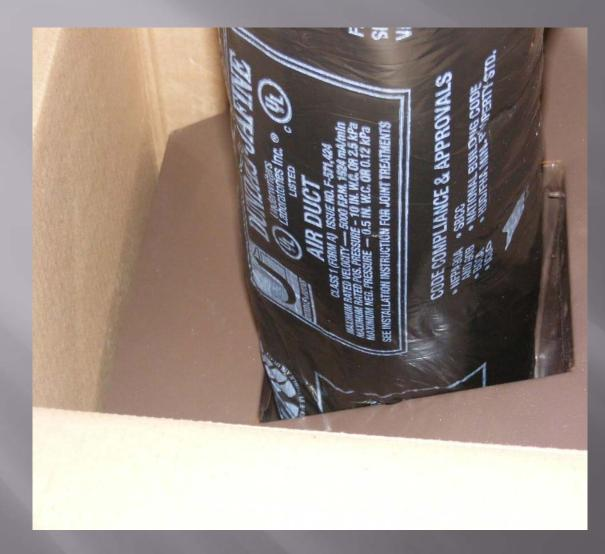
Insert the insulated sleeve over the duct and into the unit, making sure it rest completely at the bottom and that no insulation is exposed.
