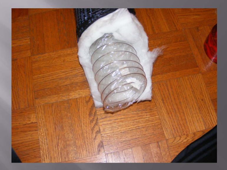
Roll the polyethylene over the insulation and between the duct, making sure no insulation is exposed.
