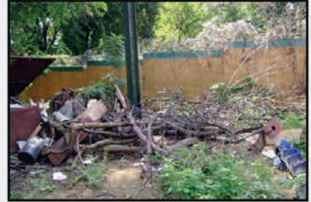
Remove debris from around buildings
