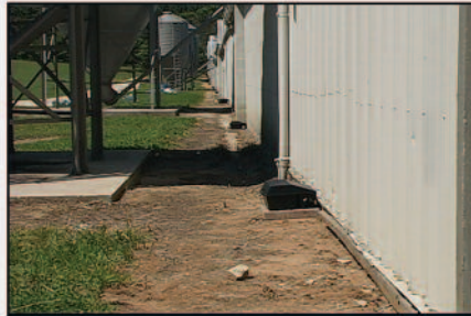
Keep a 3-foot sterile zone around buildings mowed or sprayed
