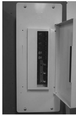
Step #3 Install New HFLCI
