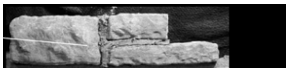
The larger stones can be leveled using two smaller stones equal to it in height.
