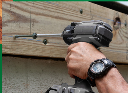
Deck Ledger Attachment
