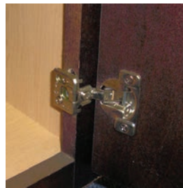
6-way Adjustable Hinges (full overlay detail)
