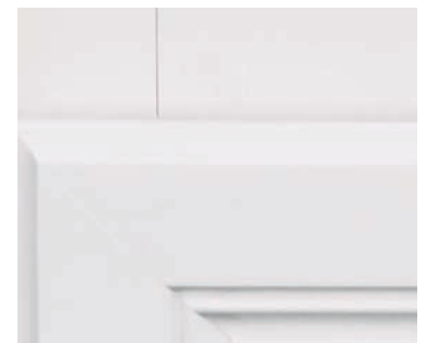
separation of frame joint
