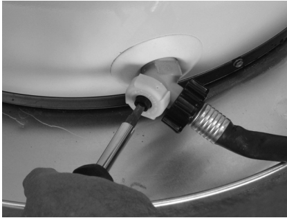
Figure 10 - Draining the old water heater.
