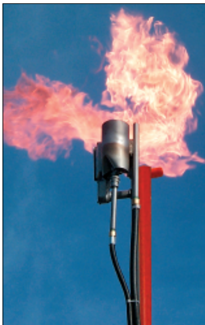
According To The NFPA (3-2.4.8 and 4-3.1), you must NOT vent LP Gas into the atmosphere.
