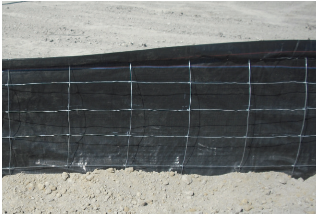
Erosion control silt fence backing.
