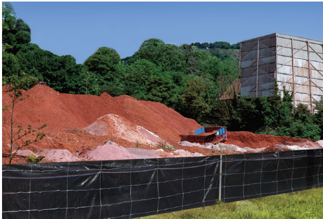
Erosion control silt fence backing.
