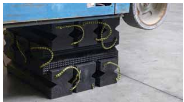
Stabilisation blocks are designed according to a system of interlocking blocks. In this photo, we see SB 002B blocks set up for a 3 stage crib application.
