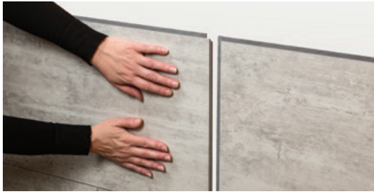
Lock tiles by sliding into joint For wet environments, use a silicone-based sealant in seams.
