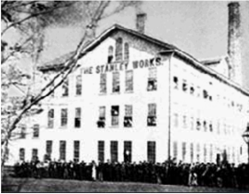
The Stanly Works New Britain, CT in 1843
