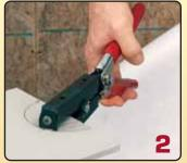
**Use Notcher to score along** marking to avoid fractures outside arc.
