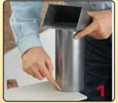
Mark the arc of outlet diameter to be removed from plank.
