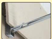
Place pair of gauges on top edge of lower plank as shown. Rest upper plank against outside face of the gauge stop to accurately space planks, and then nail upper plank approximately 18" (46cm) away from gauge as shown at top of page at right.
