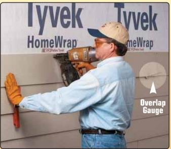
Using the Facing Gauge while nailing across the width of the plank assures greater accuracy of the desired exposure and guards against sagging. The Malco Overlap Gauge is used here like an extra pair of hands to prop up one end of the plank for one-person application.
