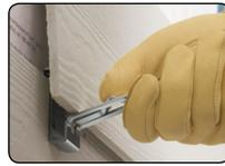
Depress thumb tab to allow plank to snap flush to wall and gauge.
