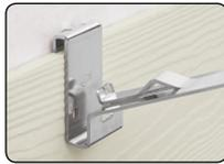
Place pair of gauges on top edge of lower plank as shown. Rest upper plank against outside face of the gauge stop to accurately space planks, and then nail upper plank approximately 18 in. (46 cm) away from gauge.
