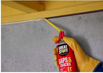
Rim Joist/Sill Plate
