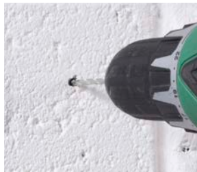
Drill a 3/16" (0.1875") pilot hole
