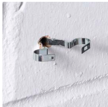
Rest Stag Clip in the pilot hole ready to accept cable(s)
