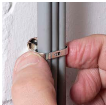
Insert cable(s) before squeezing the smooth head
