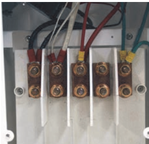
Copper Busbar with Ratings from 250 to 500 A
