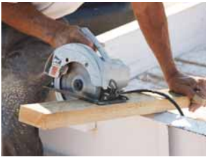
Construction Site Application
