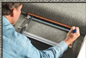
FROM TOP STAIR - STRETCH
