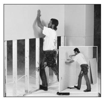
**Glue.** Even strong constructiongrade panel adhesives must be reinforced with nails and screws. Make sure the framing surfaces are clean and free of contamination. Apply adhesive, following the manufacturer's instructions. Then use nails or screws, spacing them 16" apart in the field of the boards.
