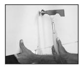
To install drywall horizontally (at right angle to the framing), start with the top board. Place together the tapered factory edge, moderately touching. Push the board firmly against the ceiling and fasten with nails or screws placed 7" from the interior ceiling angle. Space all nails 7" apart and screws 12" apart.
