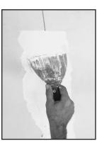
Popped nails. Press the board firmly against the framing member. Drive and dimple a new nail about 1-1/2" from the popped nail. Then drive the first nail below the surface of the board. Cover the dimples with joint compound.
