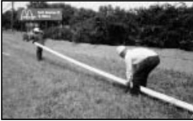
**1.** Distribute Multi-gard sections along the sides of the trench with male ends pointing towards starting vault entrance.
