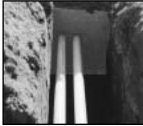
**2.** Remove protective cap and install Multi-Gard terminator on male end. Install first section into vault opening or enclosure making sure the print line is on the top stating "INSTALL PRINT LINE UP." (See next page for terminations.)
