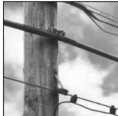
**Aerial Hanging:** Figure-8 Duct has a choice of two integrated mounting strands that attach directly to poles using 3-bolt mounting clamps, and Carlon stripping/cutting tools.
