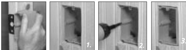
Our Low Voltage Adjustable Brackets simplify installation with tile, paneling, or stucco to save you time and effort. Just use the quick-mount bracket to clip it to the stud (1), add a screw for extra support if you want it (2), then use the adjustment screw to accommodate wall thickness (3). Also available in a two-gang version.
