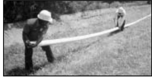
**3.** Each consecutive 20' section can now be placed by inserting the male end into the gasketed belled end 1/2" to the gasket depth. Make sure the print line is upright. (If not, rotate the outer duct until it is.) Now push the sections together with a firm push until belled end seats against insertion line.
