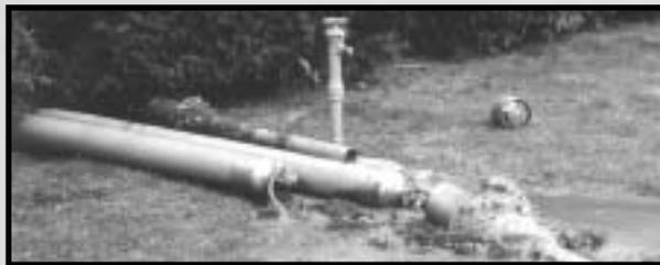
*Horizontal Directional Drilling was the preferred method of installation because it minimized any disruption to the island's pristine environment.*
