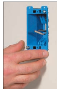
Place Box in Wall
