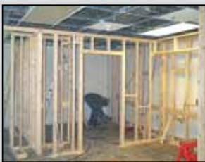
Partitions on concrete
