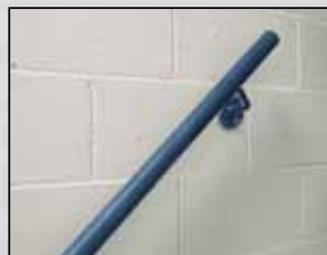
Stair rails on block
