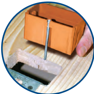
Install clip over subfloor.
