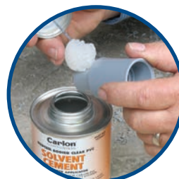
Apply a uniform coat of cement.
