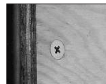
Plywood to steel or wood studs.
