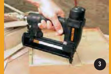
18-gauge brads fastening quarter round
