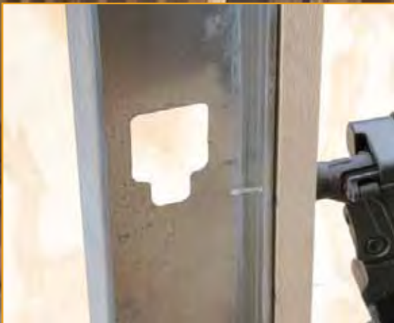
N66C Applying C4DCSBALG Ballistic Point Nail to steel stud
