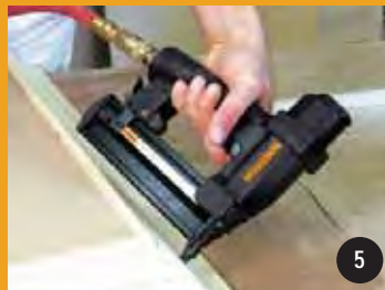
18-gauge brads applying trim
