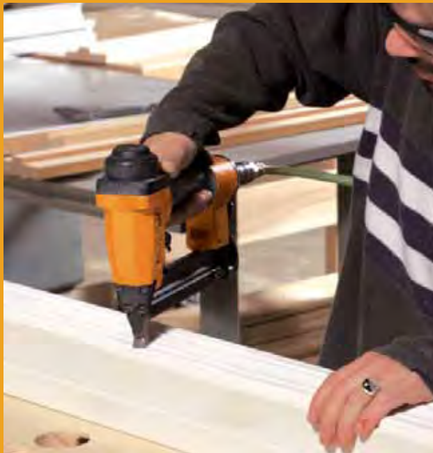
Applying 18-gauge brad to door casing
