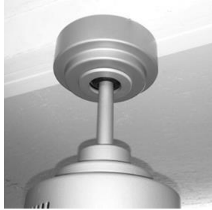
Photo 9: Complete hanger assembly
