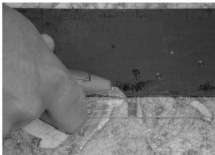
For those installers who straightedge and butt seams, the straightedge should be positioned so that the cut is made 1/8 away from the end of the pattern match indicator on both sides of the seam. This will assure proper match at the seam.
