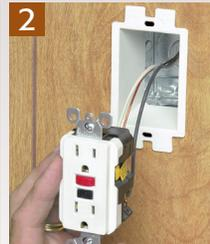
2 Attach wires to receptacle. Tighten screws for a level, fully supported, code compliant installation.
