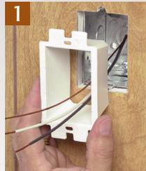
1 Pull wires through. Press the BE1 firmly into the electrical box.
