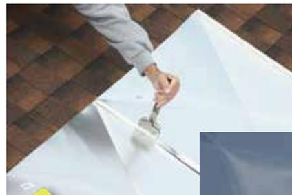
Wide Flange Pliers Metal Bender (page 75 for more information) being used to crimp panels together.
