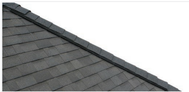
Hip Ridge Vent Installation
